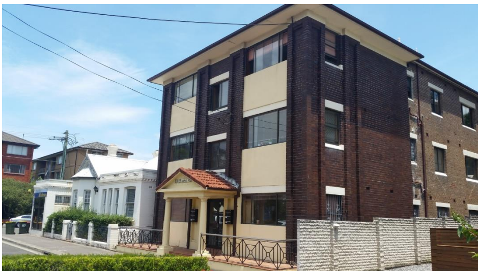
Figure 18 – Properties adjoining the site to the south
